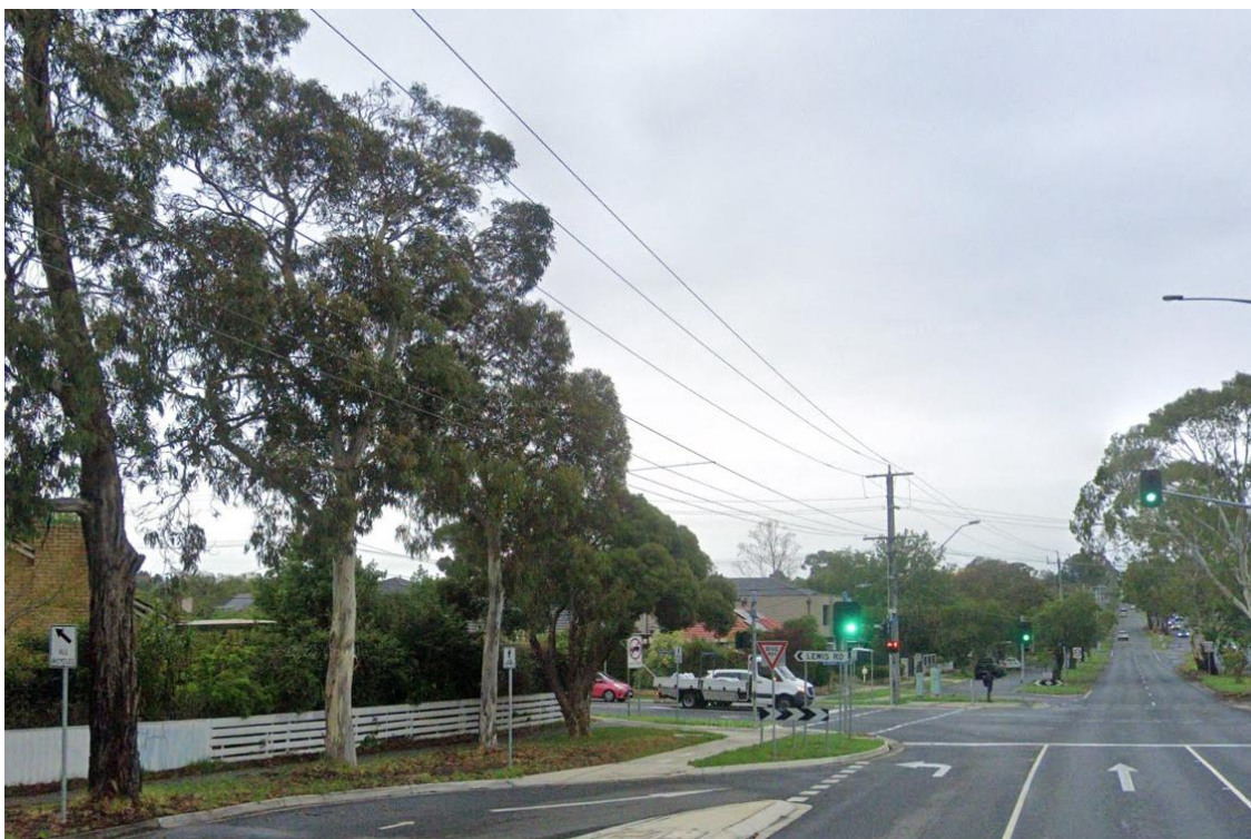
Boronia Rd/Lewis Rd – Lights at intersection 2022.
